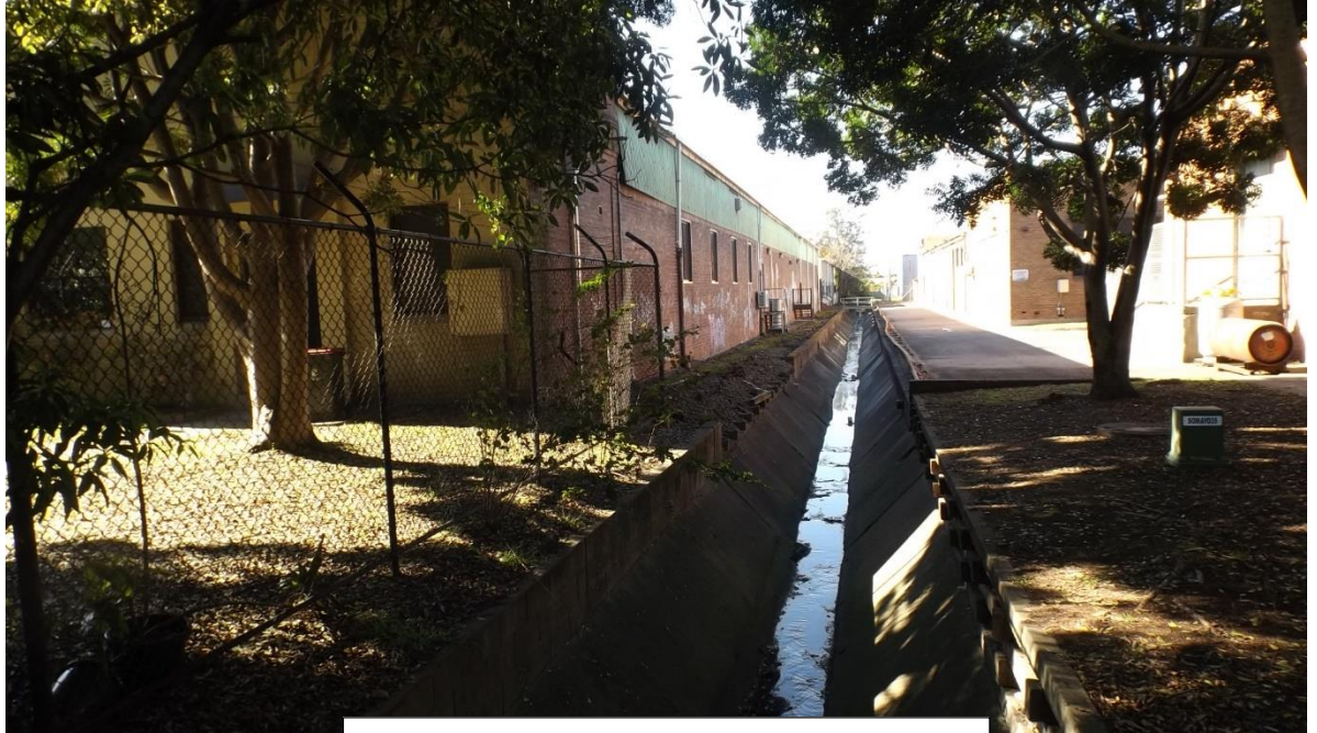
View looking east along stormwater canal immediately north of University grounds and south of U-store.
