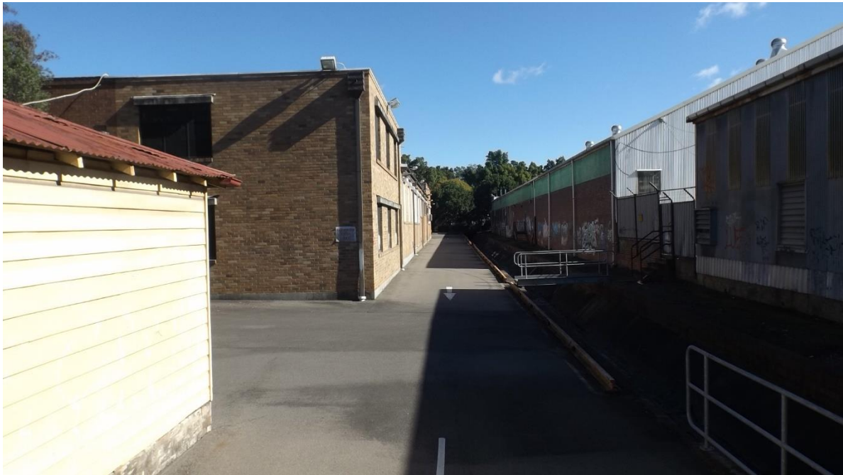
View of canal between u store and University buildings looking west towards Frith Street
