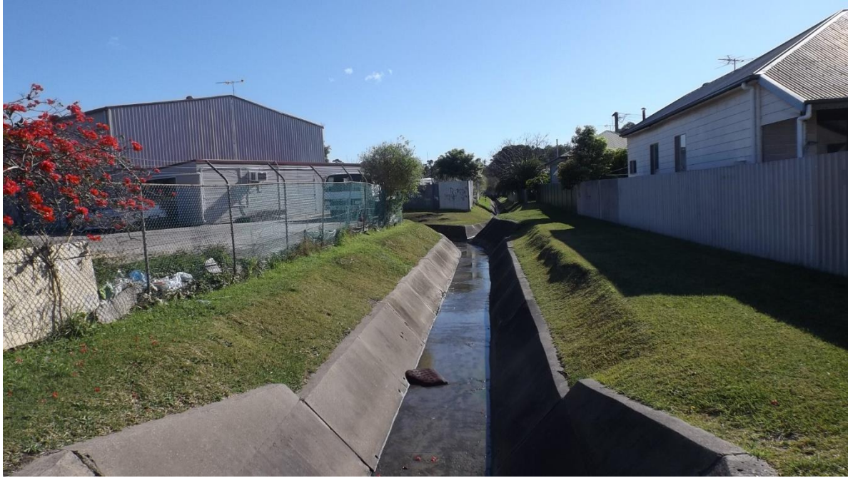
View looking north along canal at east of 14-16 Gavey Street
